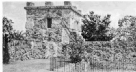
The fenced-off area is where Ed quarried his stone
